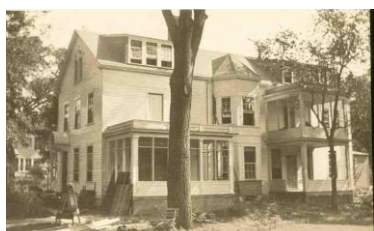
1914 The Cottage under renovation
